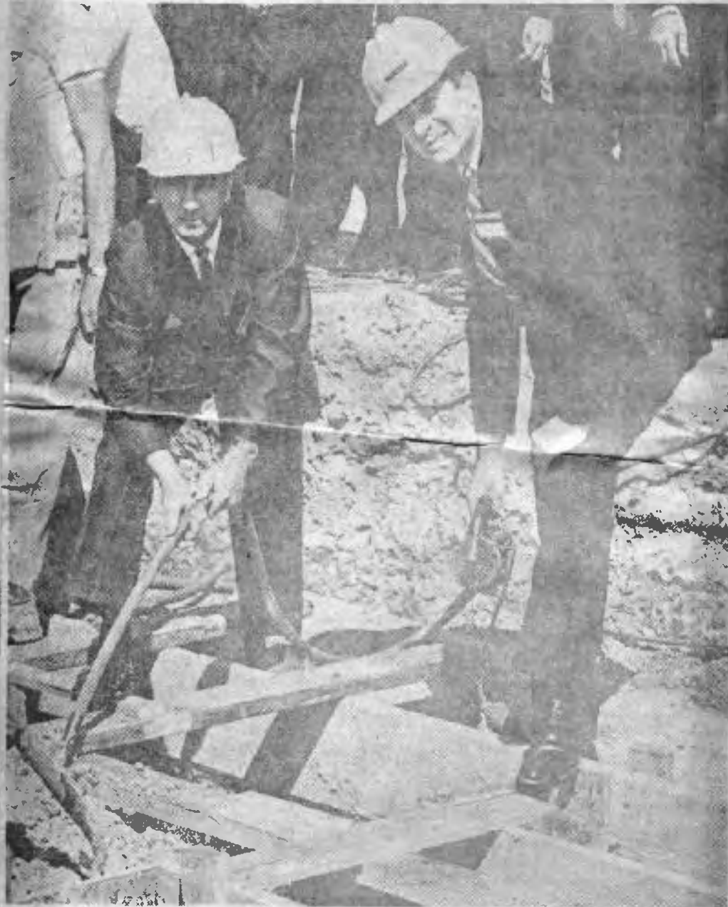
WHEELING VILLAGE PRES. Ted Scanlon and Skil Corp. Pres. John W. Sullivan initiate construction of Skil's new Wheeling power
