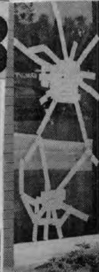
LARGE WINDOWS AT THE front of the Cartriseal plant in Wheeling are being repaired following Monday morning's devastation. Eight windows valued at $400 each were
